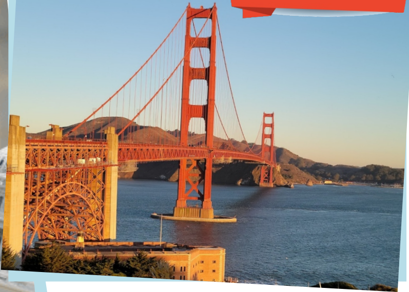
Golden Gate Bridge
